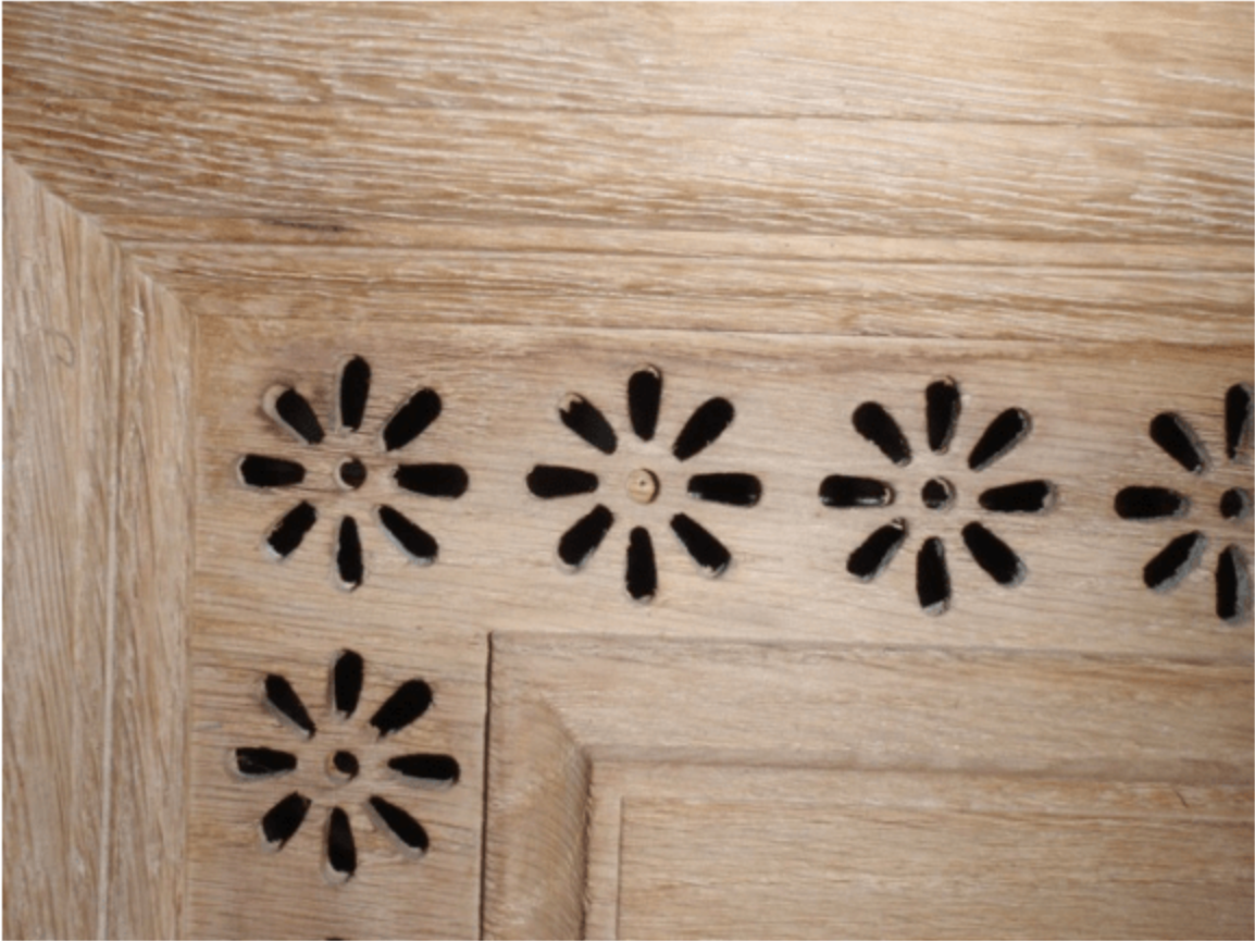
Additional example of holes not drilled through. Again no even application of staining.
