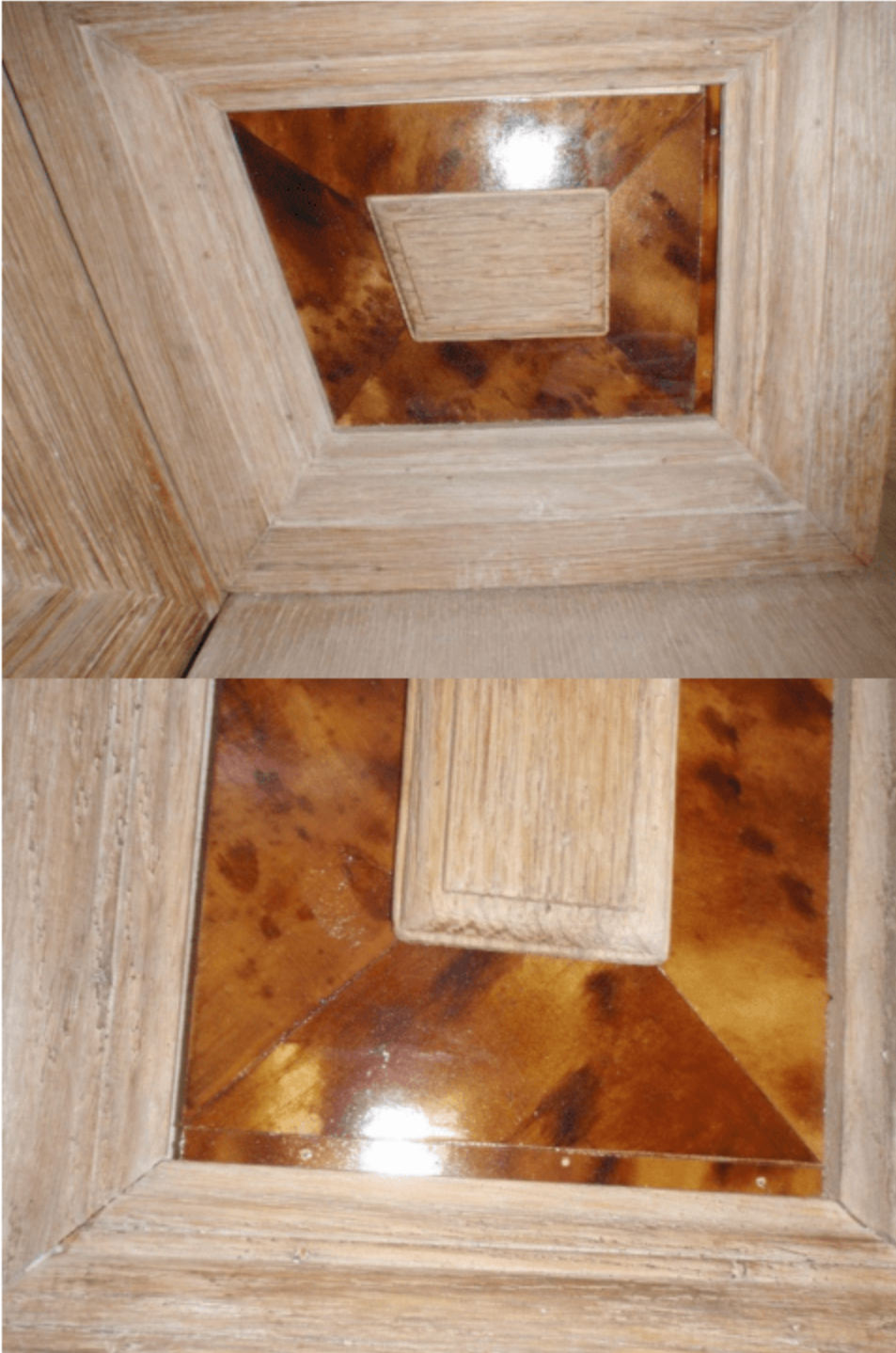
Patchwork tortoise shell. Tortoise shell not completely covering in areas (see top picture). Pin holes in tortoise shell. Surface of Tortoise shell blemished. Color finish on wood looks incomplete. Rough and pocked surface of wood. Stain color unevenly and incompletely applied.
