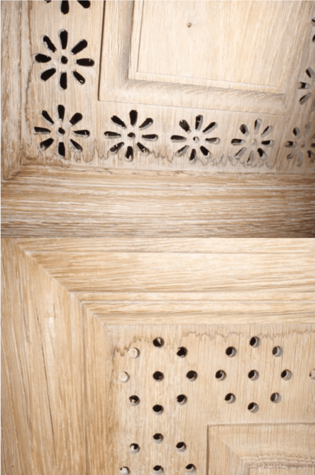
More examples of holes not drilled through and sanded and uneven application of stain appearing like water stains.
