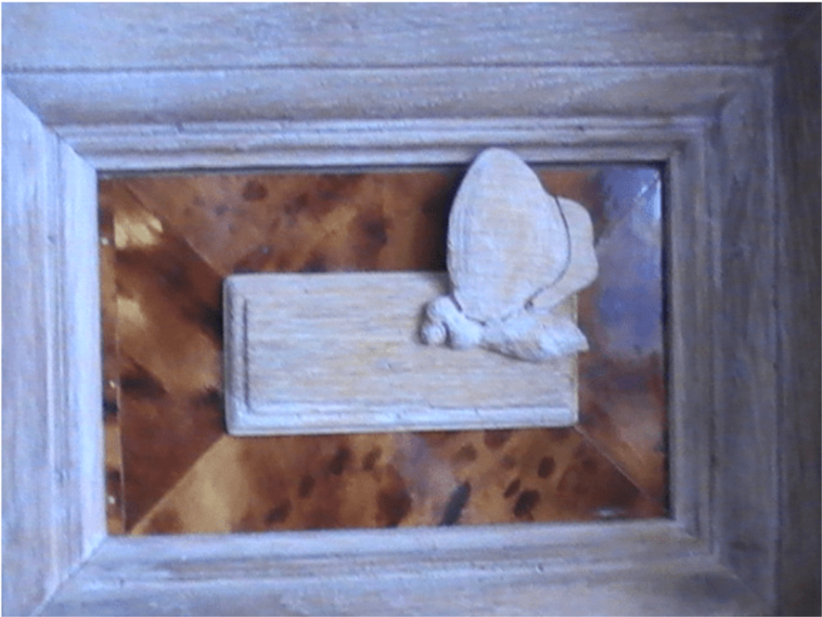
Larger picture of shoddy workmanship. Tortoise shell surface unclean. Patchwork tortoise shell. Butterfly unfinished with wood putty still evident. Rough wood surfaces and edges. Uneven application of color. Unfinished appearance.
