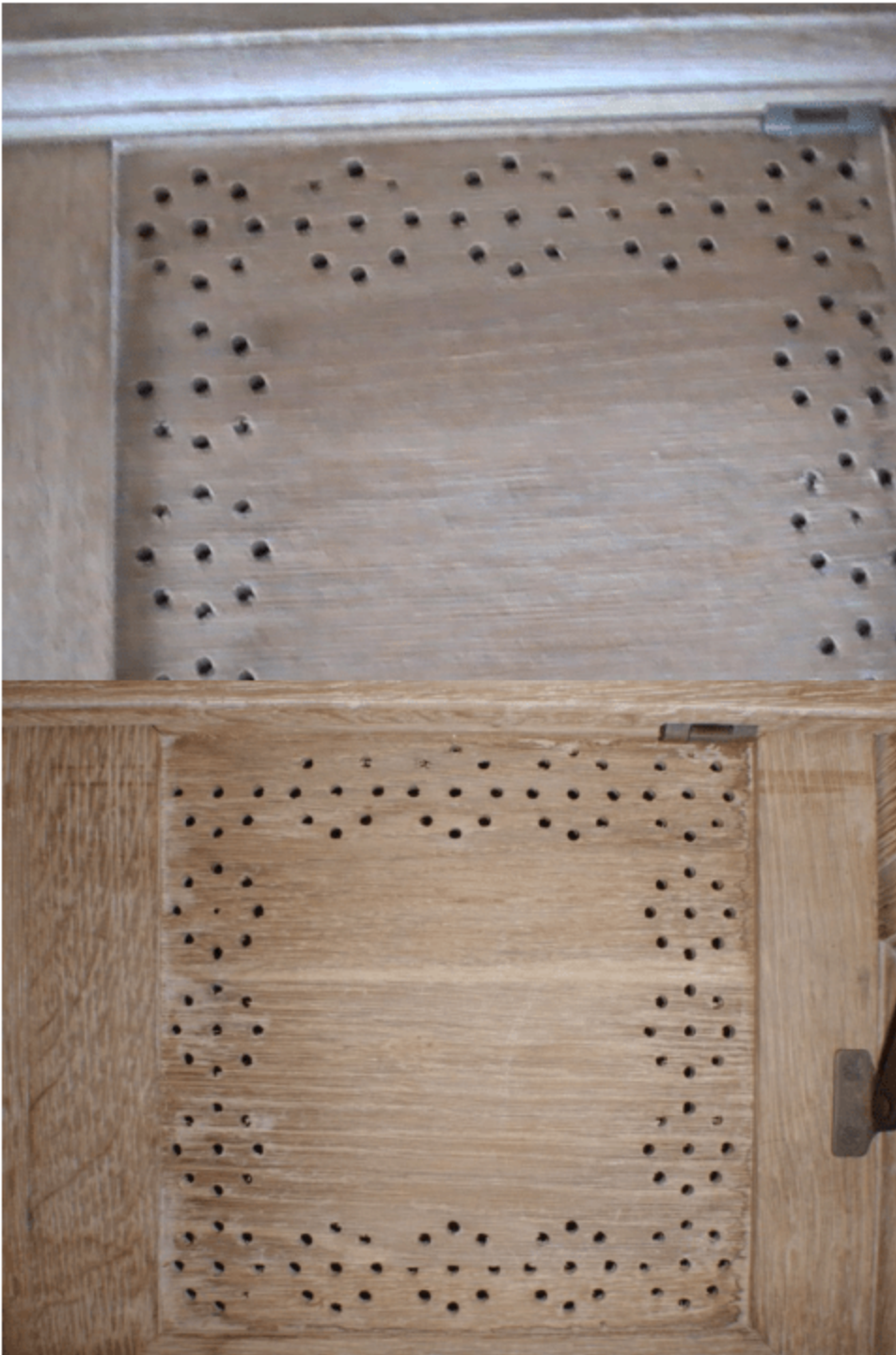
Uneven application of stain. Water stained appearance. Holes not completely drilled through or sanded.
