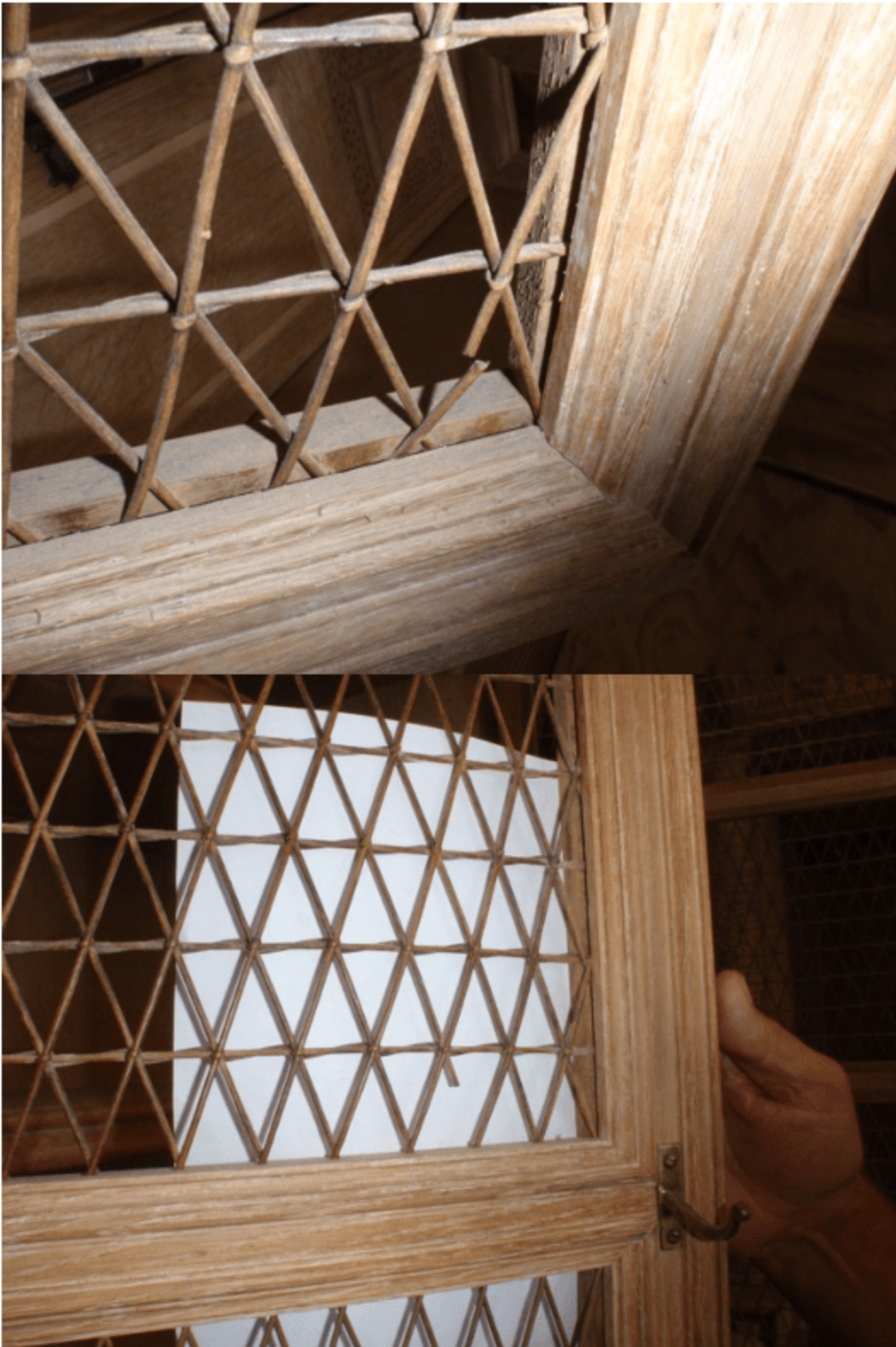
Examples of broken mesh work on cabinet doors. Poorly finished wood. Rough splintery wood. Uneven application of color.
