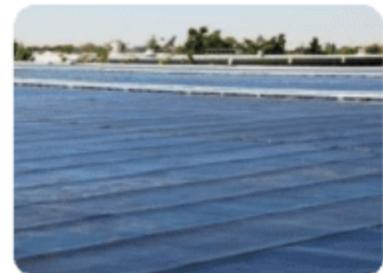
The thin-film photovoltaic (PV) system covers 95,000 sq. ft. of rooftop, and is expected to generate about 667,000 kWh per year with a peak rating of 468 kW. The system supplies approximately 13% of the building's electricity needs.
